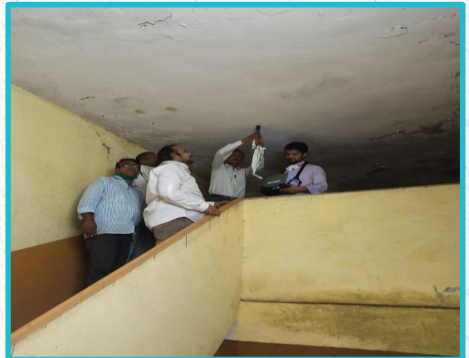
Corrosion meter Test on Slab
